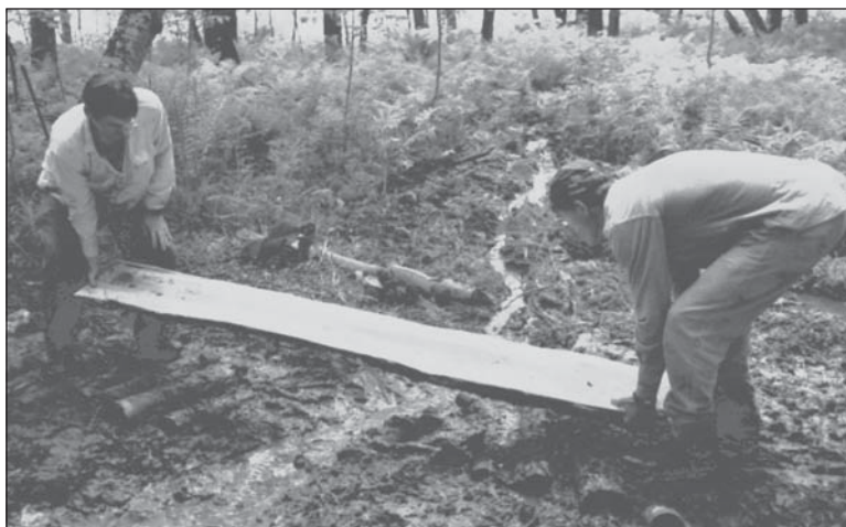
National Trails Day—VMBA volunteers spent a total of 30 working hours building "corduroy" on the Cotton Brook Trail. VMBA has a Cooperative Agreement with the Dept. of Forest, Parks & Rec. to maintain the Cotton Brook Trail in Mount Mansfield State Forest.
